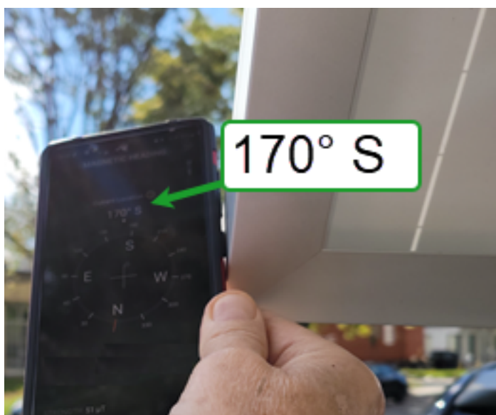
[Figure 12] Aiming the panel to True South with a compass app
